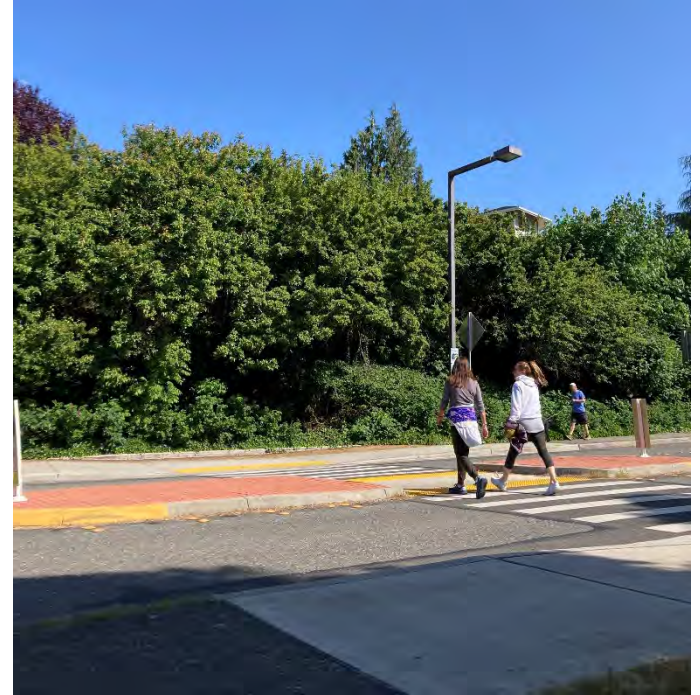
Photo of pedestrian crossing and median island.
