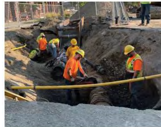
Construction Crew replacing water main on Post Street.
