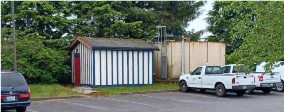
Figure 11: Pump House from Site Assessment
