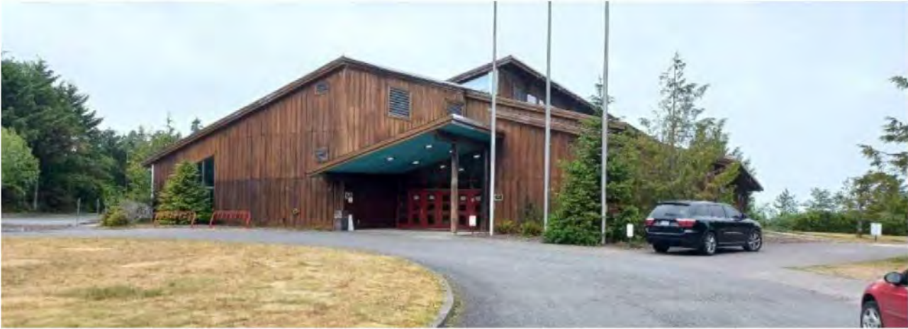
Figure 10: Akalat Building Front from Site Assessment
