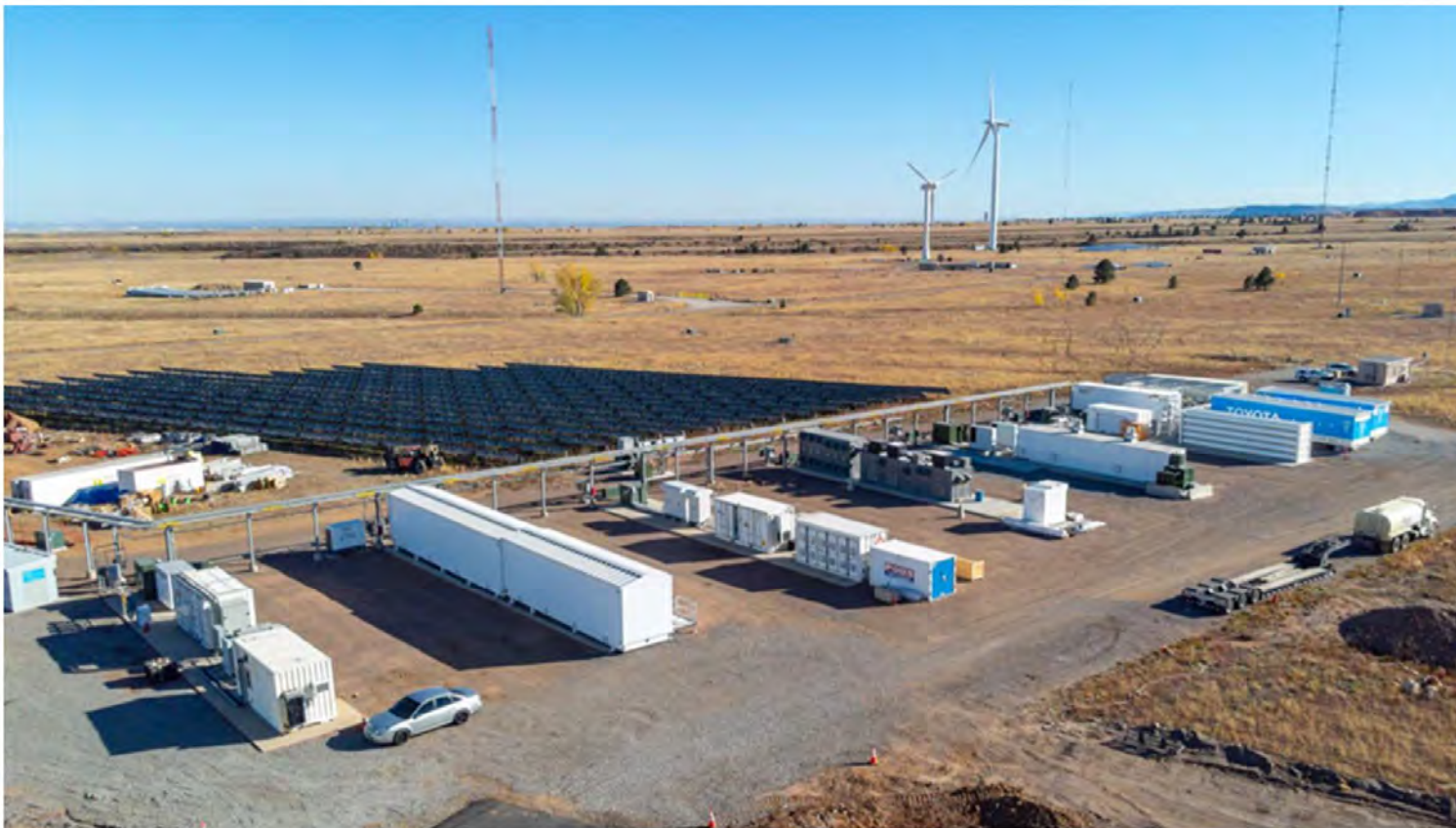
The Advanced Research on Integrated Energy Systems (ARIES) capability at NREL is fully equipped to emulate energy systems of any design. ARIES enabled NREL to replicate and receive real-time data from the electrical system of Cordova, Alaska, to develop resilience and advanced grid visibility applications. Photo by NREL
