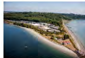
West Point Treatment Plant Photo credit: King County, WA
