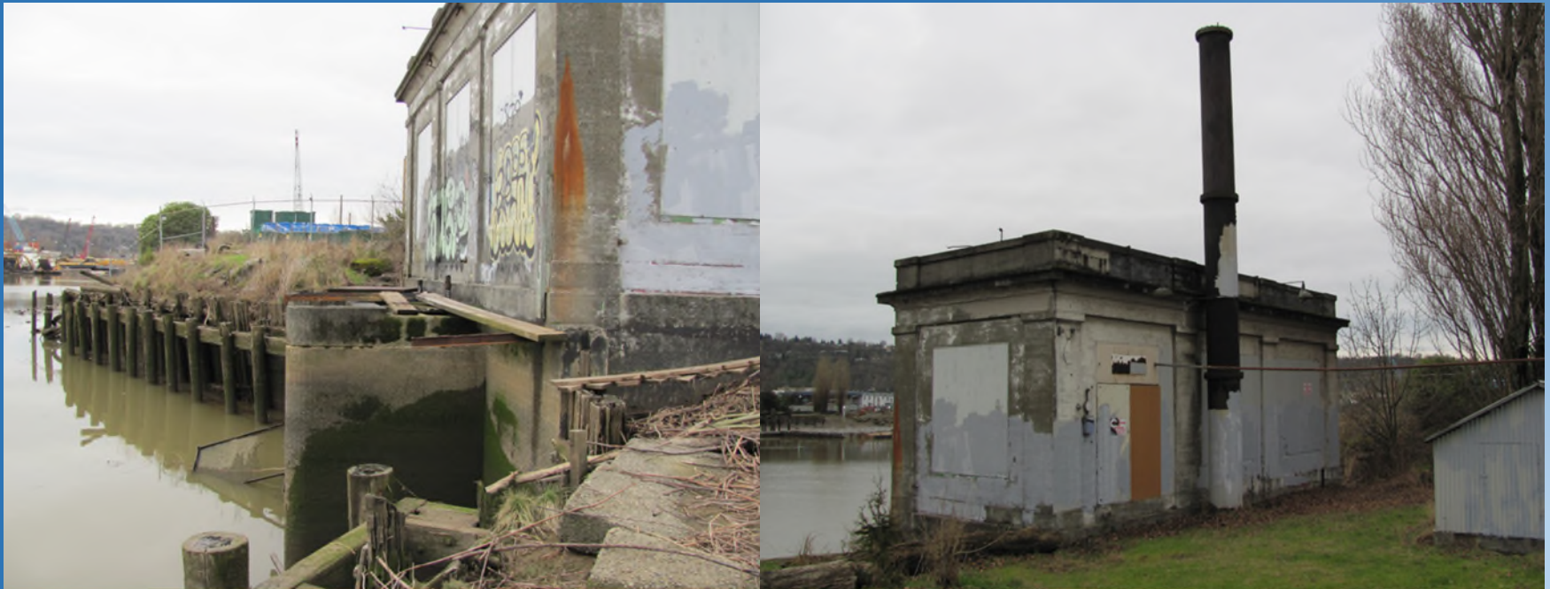
Georgetown Steam Plant Pumphouse – Seattle Duwamish Waterway
