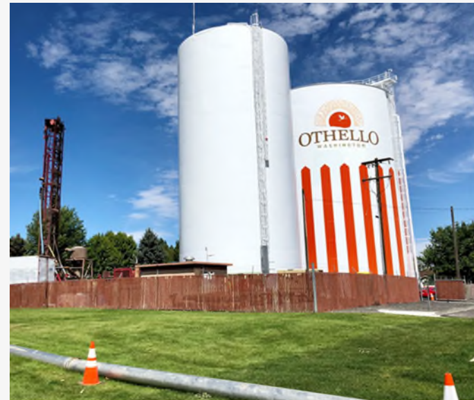
City of Othello ASR pilot project (2020)
