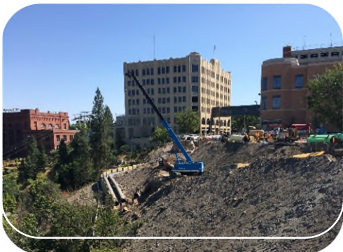
Combined Sewer Overflows (CSO)
