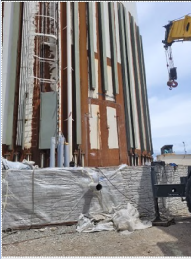
During Retrofit Construction
