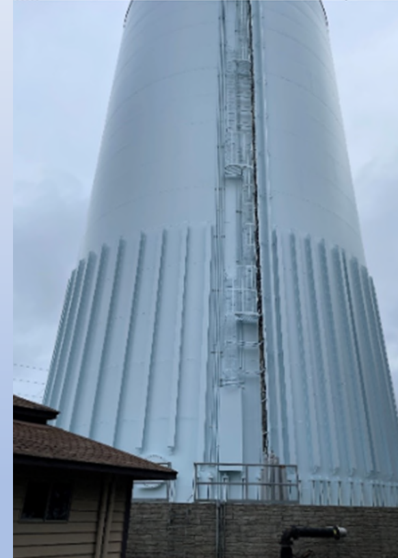
After Seismic Upgrades
