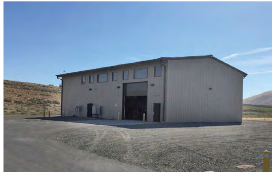
Entire plant fits neatly inside one building!
