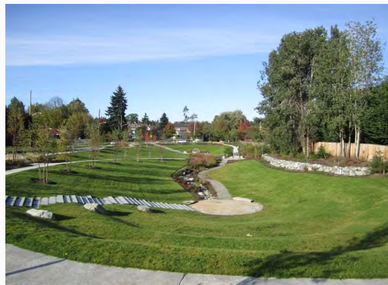
Seattle Madison Valley Stormwater Park
