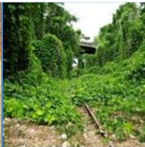
Other environmental contaminants
